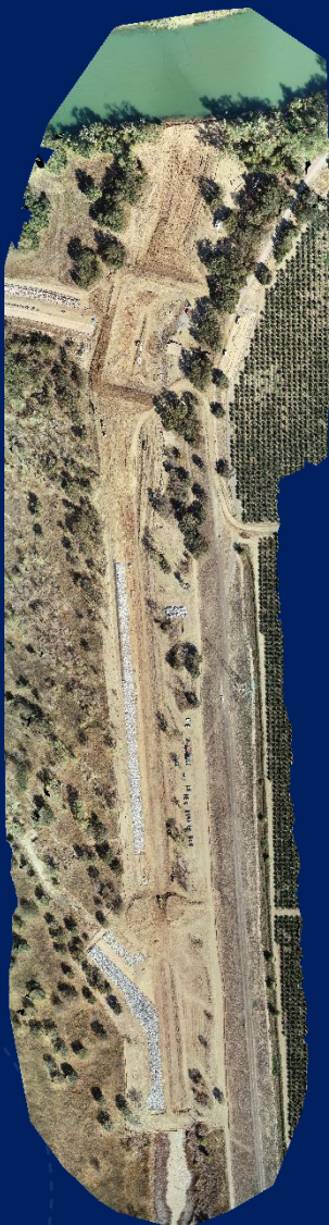
Big Notch Project: Construction Monitoring
